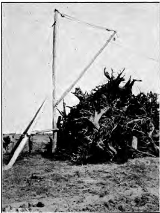
Fig. 62. Light Derrick Used on Tract 5
